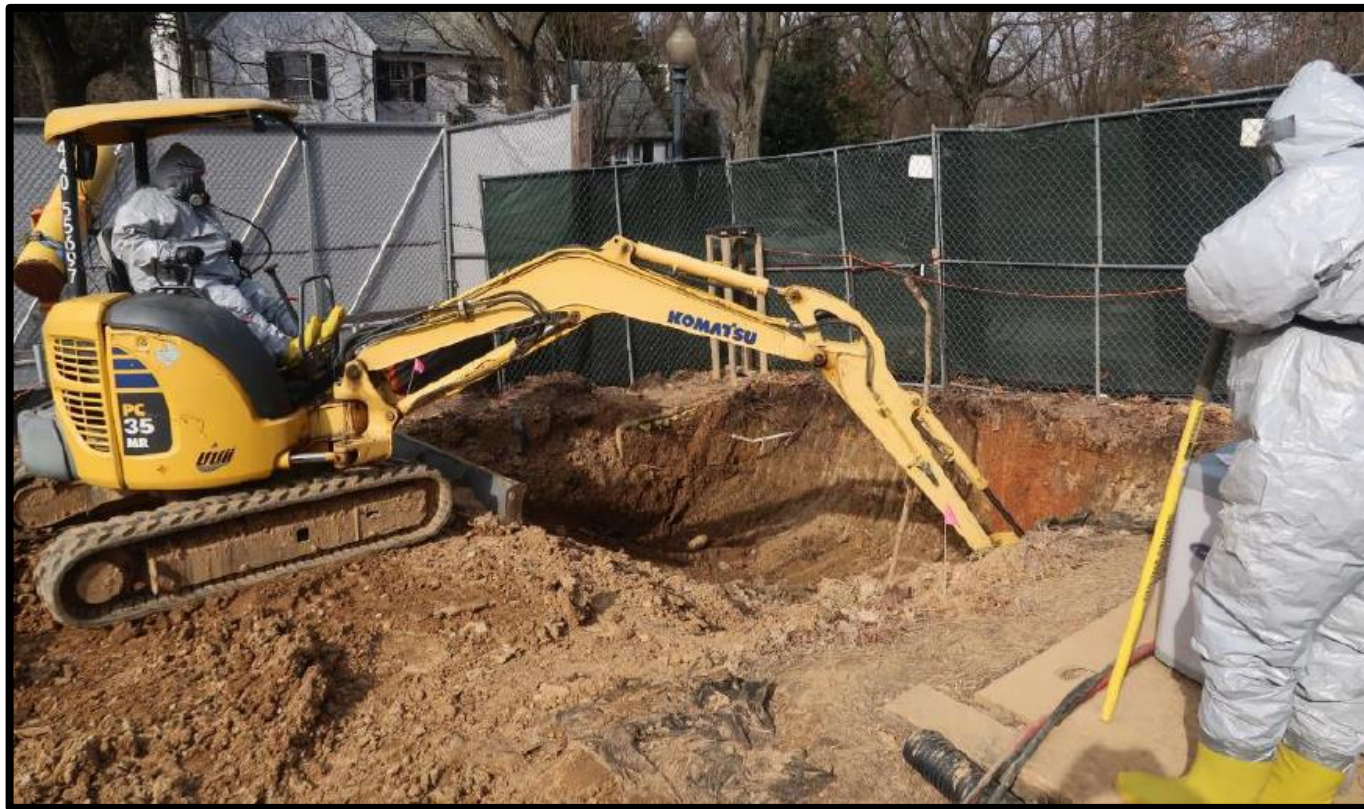
Over-excavating in Area 3
